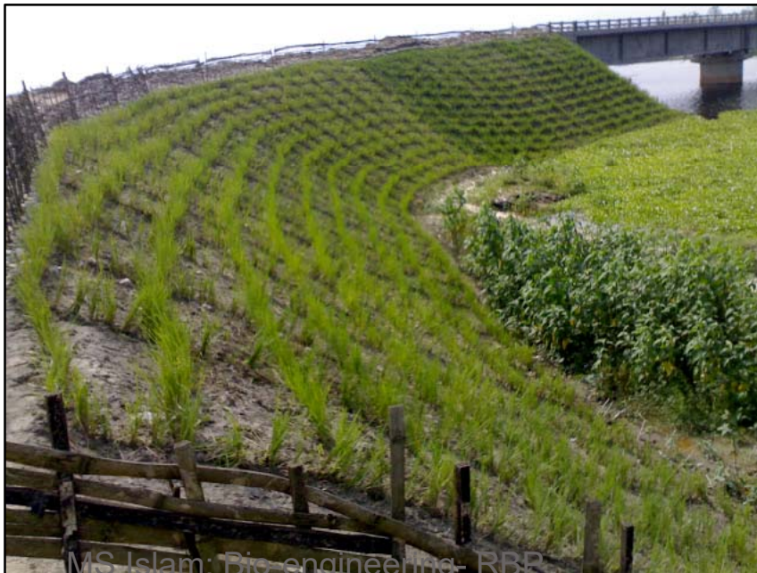
Bridge Abutment Stabilization, Assam, India
