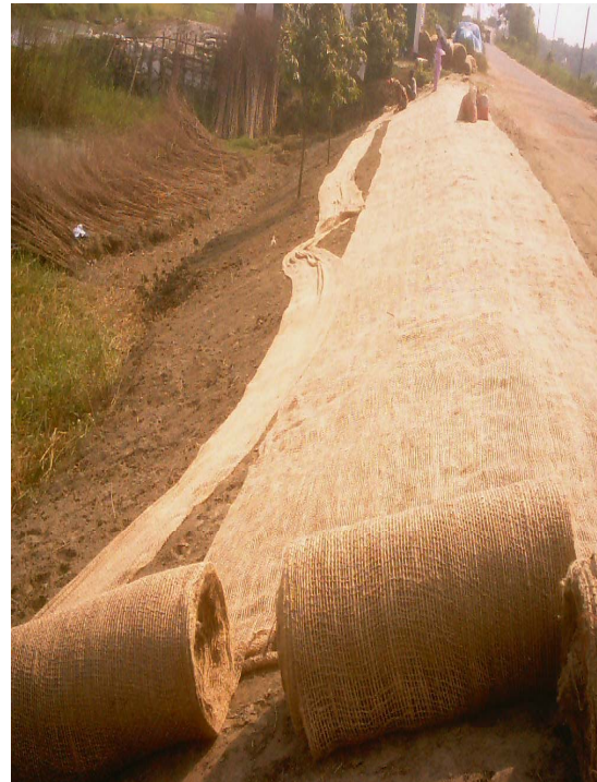
B) Laying and fixing of geo-jute
