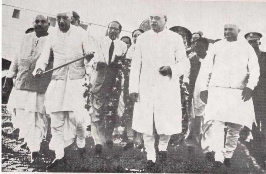
No. 6. The Prime Minister inspected Dibrugarh erosion on 4th September, 1954.
