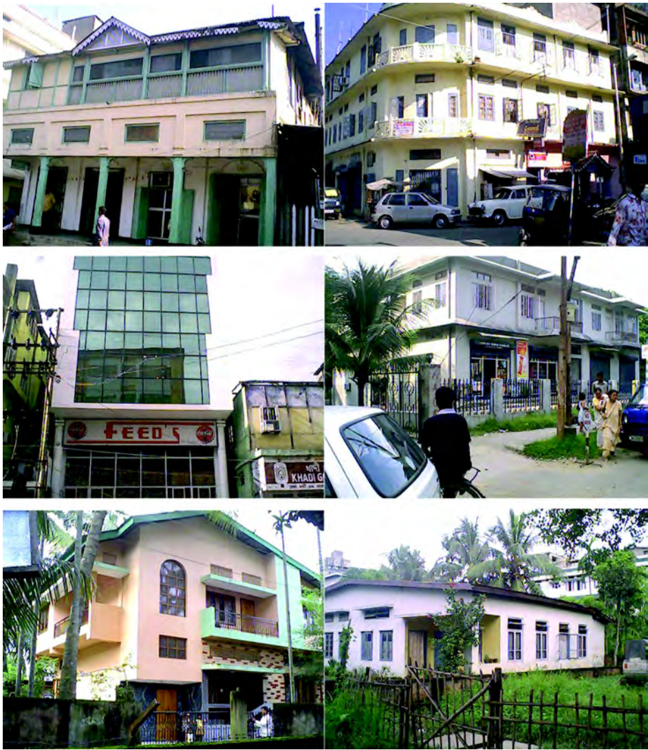
Figure 8.1 Existing building typologies in Guwahati urban area
