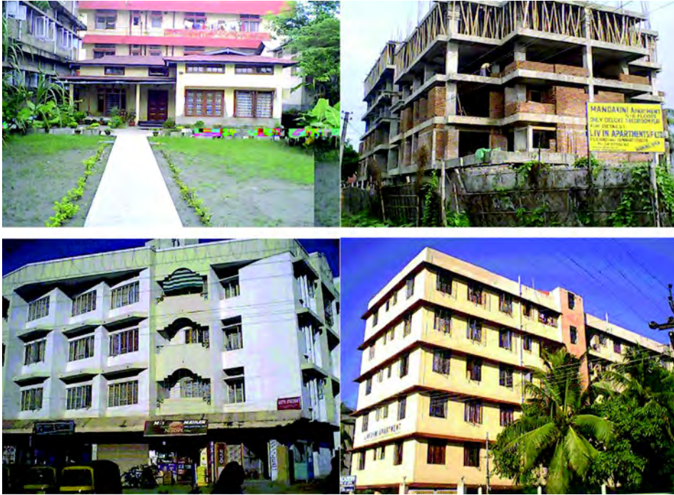
Figure 8.2 Existing building typologies in Guwahati urban area
