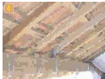
In wind speed area use galvanized metal straps along with 2 nails. Pre-drill pilot holes.
