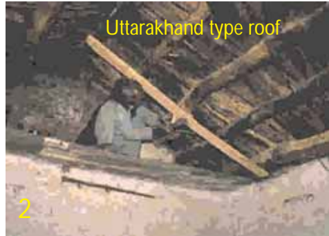
2. Using two nails at each end install a 100mm (4") x 25mm (1") strut (plank) on the underside of purlins adjacent to their ends.
