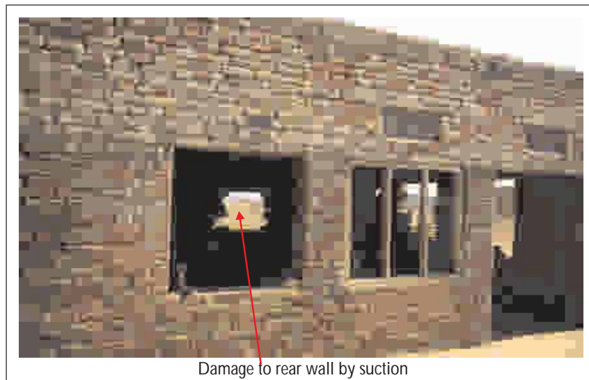
Collapse of wall and damage to roof
