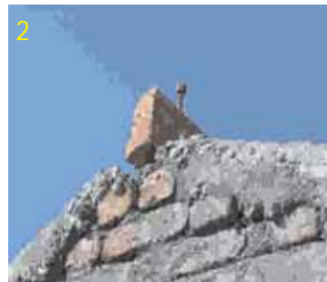
Once concrete becomes hard place timber beam with a through hole over the bolt and place a washer and a nut to anchor it down.
