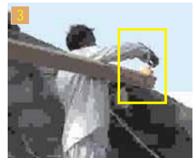
Once concrete becomes hard place timber beam with a through hole over the bolt and place a washer and a nut to anchor it down.
