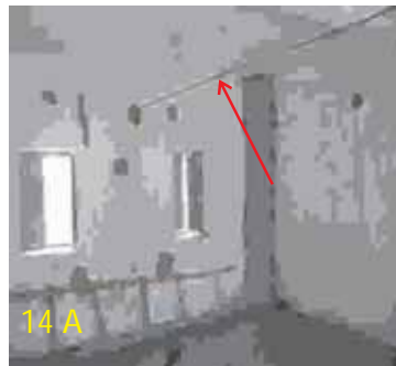
14.A Tie rod must be installed level from one wall to the opposite wall going clear through a conduit placed in both walls and through the belts.
