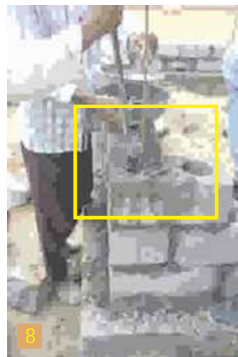
Use solid blocks with key-hole or hollow blocks with a slot keeping reinforcing rod in the center of the cavity, and fill it with micro-concrete in 450mm (18") lifts.
