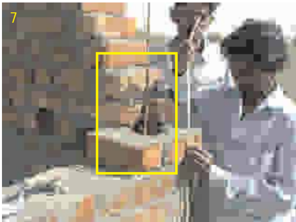
Use solid blocks with key-hole or hollow blocks with a slot keeping reinforcing rod in the center of the cavity, and fill it with micro-concrete in 450mm (18") lifts.
