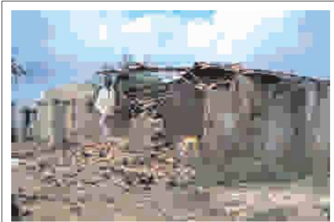
Collapse of wall and damage to roof
